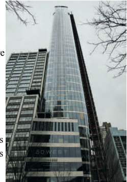
50 West is expected to be ready for partial occupancy at the end of the year. Photo: Carl Glassman/Tribeca Trib
